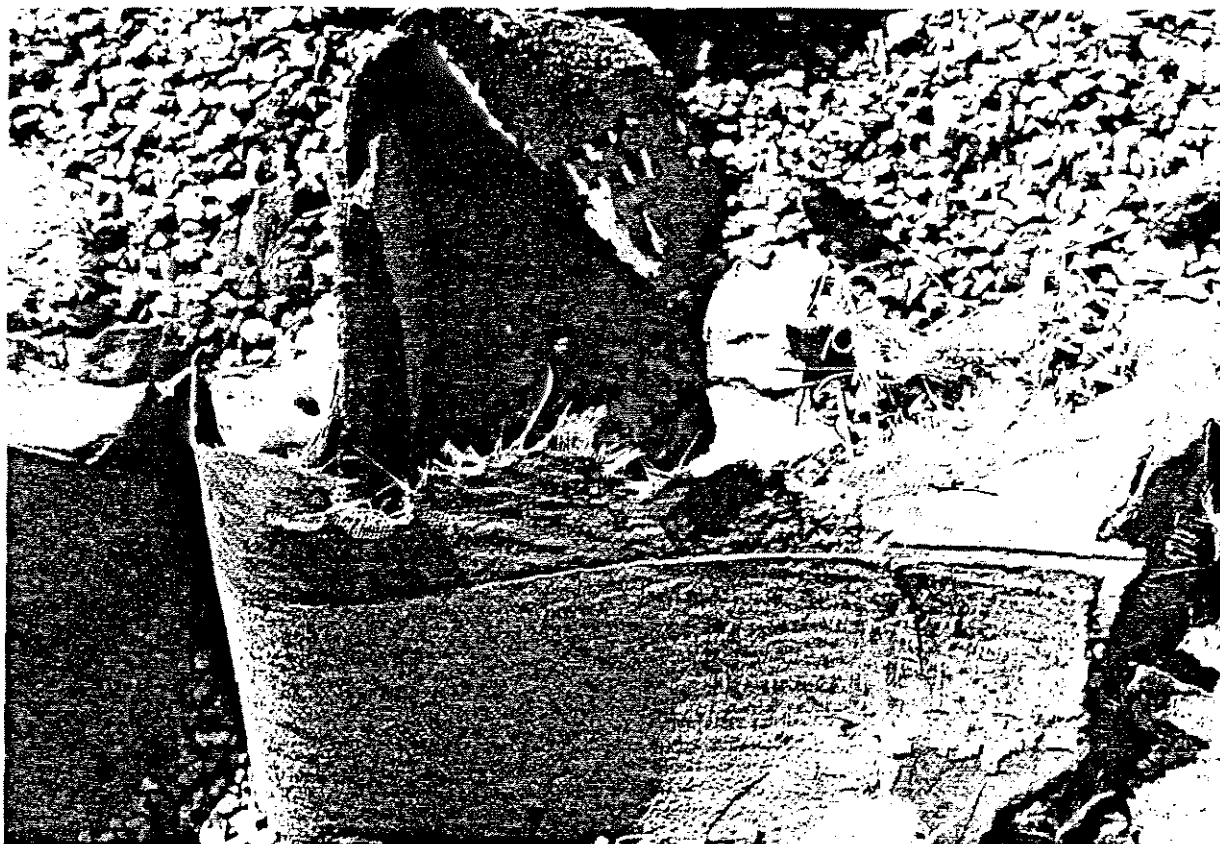
Figure 3. Asphalt roofing felts which are in poor condition. Notice the fibers protruding along the edge of this roofing felt.
